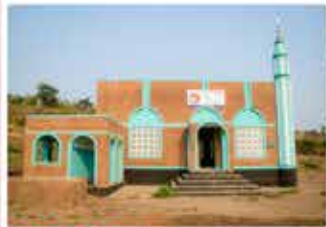
Machinga Masjid Malawi Construction
