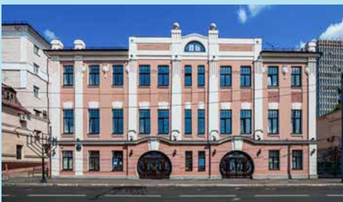
Just over a hundred years old, this synagogue was returned to the Jewish community in 1996 and has since been renovated and is now in use.
