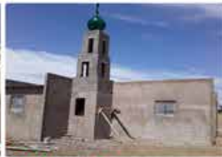
Cofimvaba New Masjid Construction
